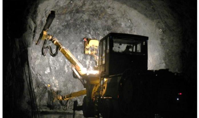
Initially a smaller 5 x 6m relief tunnel was conventionally blasted in the top middle section of the larger tunnel excavation.
